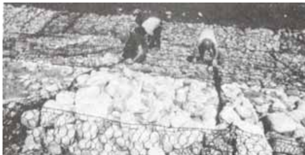
Exhibit XIII .6 Wire Enclosed Rock Riprap
